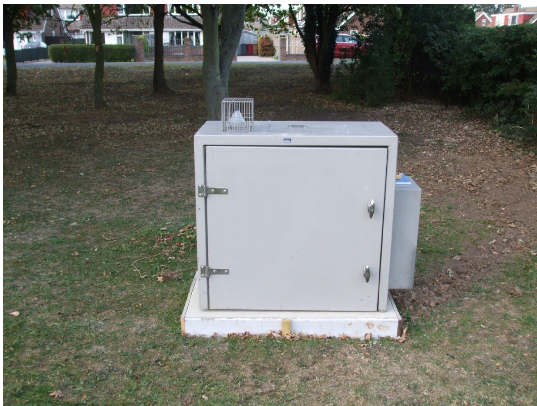
Figure 4: The enclosure containing the gas analyser located at the side of the A160 dual-carriage way.
