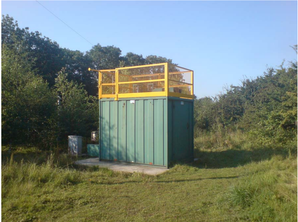
Figure 2.3a: A photo of the Low Santon TEOM monitoring station, towards the southwest.
